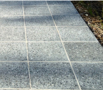
Name: Pebblecrete Material: Concrete Finish: Honed Size: Varies (Refer Landsacpe Plan)
